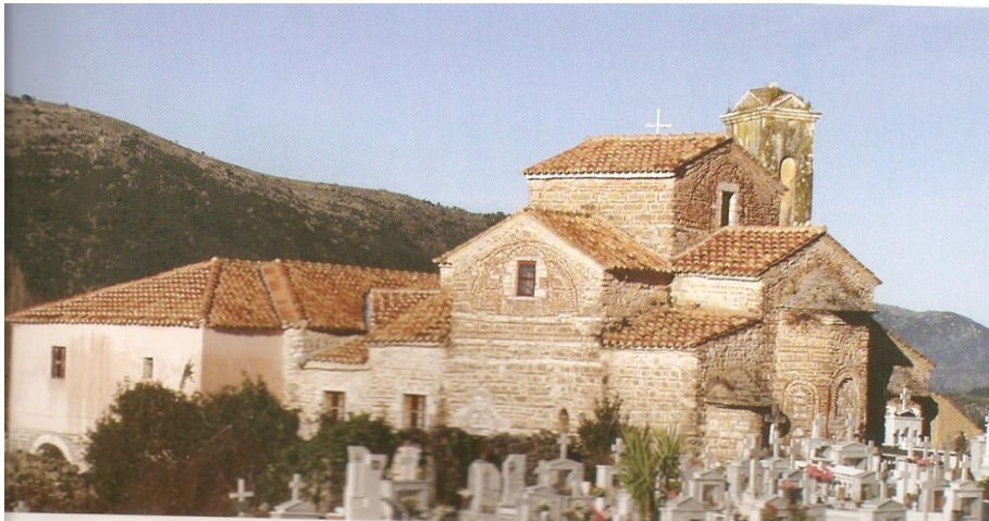
Fig. 31. Epirus. Paramythia. Church of Megali Panayia. Troullokamara on the roof.
