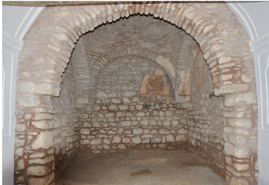
Fig.24. Mesta. Church of Ayios Ioannis Prodromos. Supports of the elliptical dome in the narthex.
